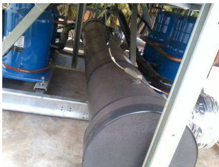
Fig. 3.26. Evaporador "Tube"
